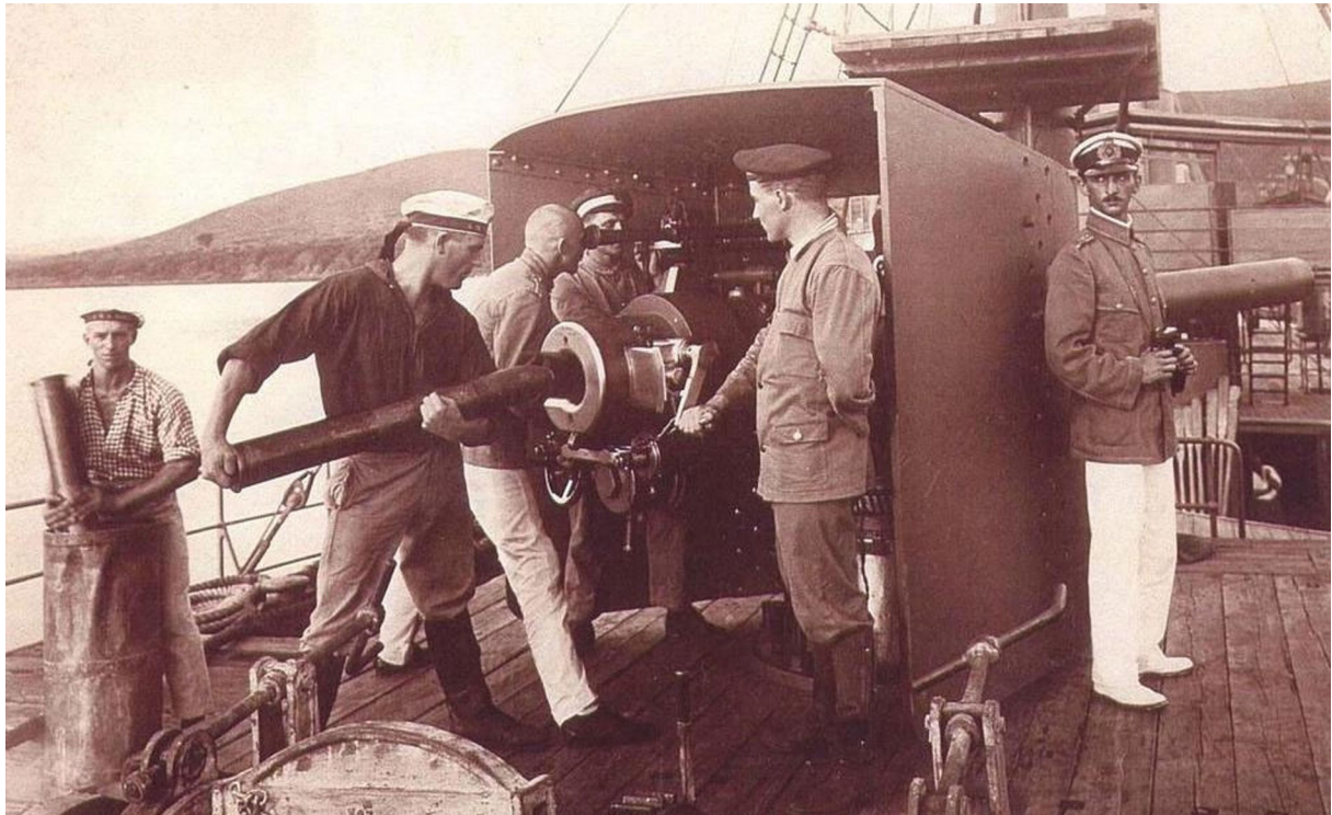
10.5 cm/40 SK L/40 onboard the german SS Goetzen in 1915 or 1916 in the Bay of Kigoma. This was the Number 6 gun salvaged from the cruiser SMS Königsberg. Note the sliding breech mechanism, typical of Krupp guns of this period. The sailor on the far left is holding a leather ammunition transfer bag.
